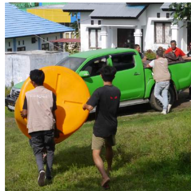
Fiber tank installation
