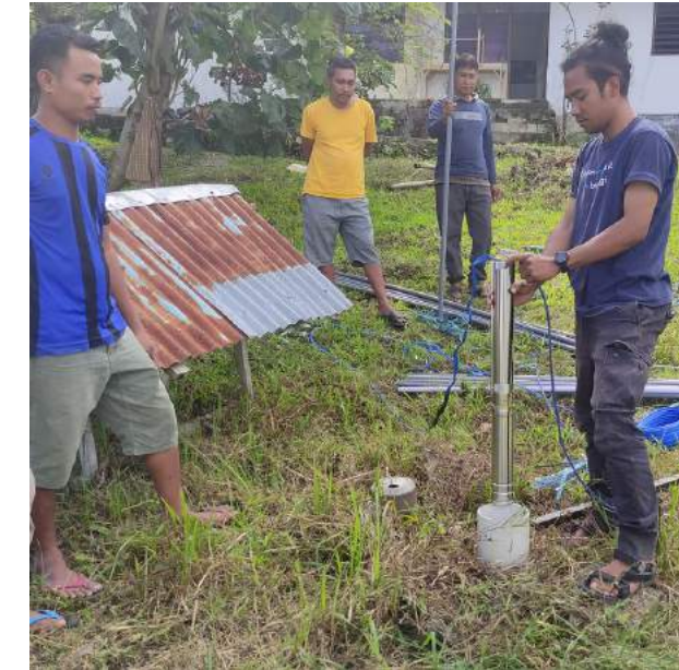
Submersible pump installation
