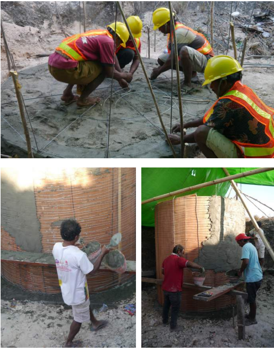
FERROCEMENT WATERTANK
